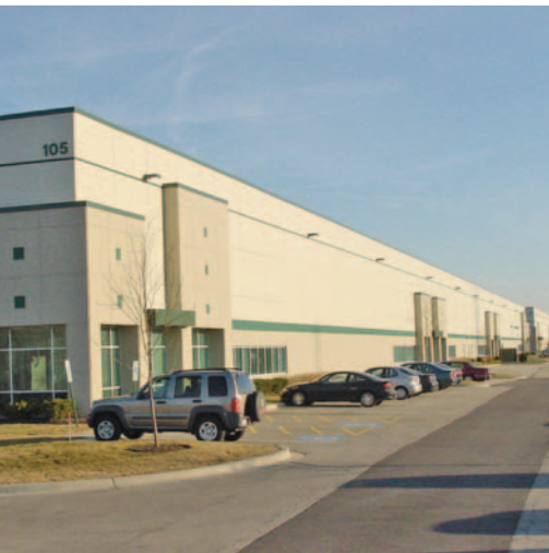
ProLogis Park O'Hare The O'Hare industrial sub-market led the area with over 5.6 million square feet of leasing and sales activity in 2003.
